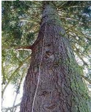
Lightning protection fitted to a 43m tall Abies procera at Eastnor Castle, Herefordshire
