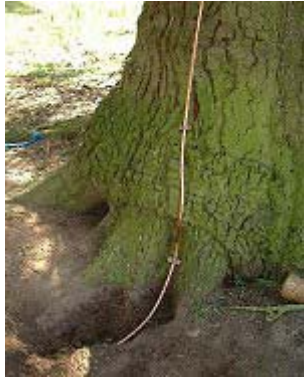
Effective lightning protection.
